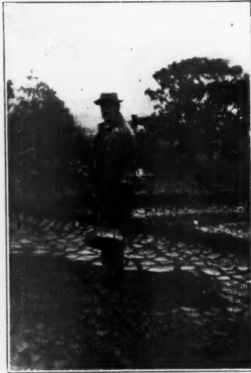
Figure 6—Removal of Sludge from Drying Beds of Pea Cannery Waste Disposal Plant, Poynette, Wisconsin
